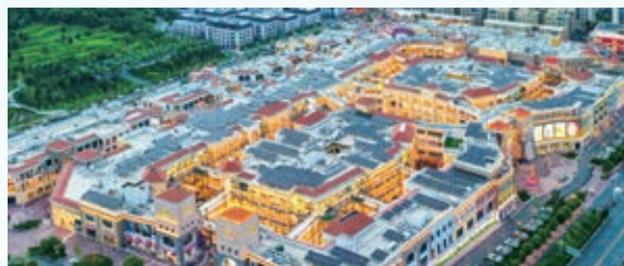
Photovoltaic Power Generation System at Jinan Capital Outlets
