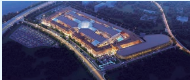
Photovoltaic Power Generation System in Hangzhou Capital Outlets
