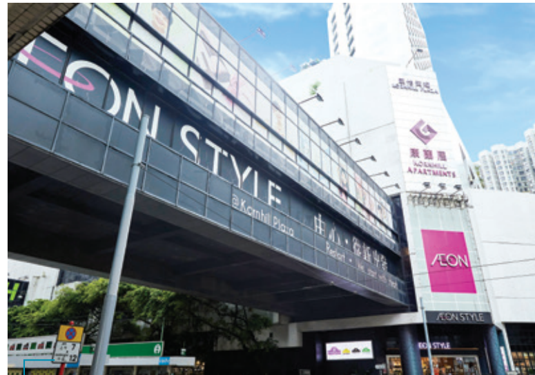
Kornhill Plaza enhanced its attraction to nearby residents with a stronger focus on the home living and wellness sectors
