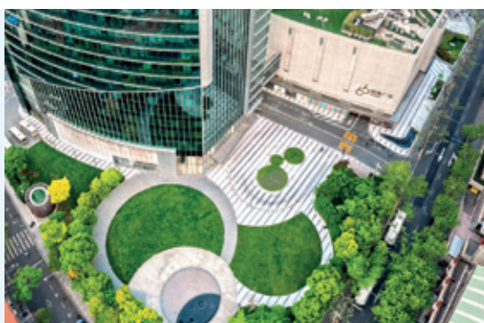
Plaza 66, Shanghai is the first operating property and the largest commercial complex in mainland China to receive platinum ratings for LEED V4.0 Existing Building: Operations and Maintenance and WELL V2 Core certifications*
