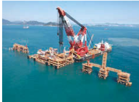
▲ Construction in progress on the jetty of the offshore LNG terminal
