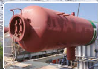
▲ L11 steam drum lifting
