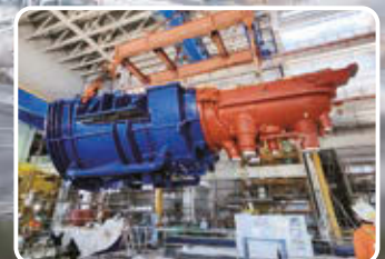
▲ Site assembly of L12 steam turbine
