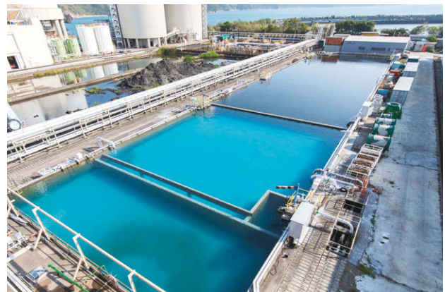
Collection pits for rainwater and reusable wastewater at Lamma Power Station
