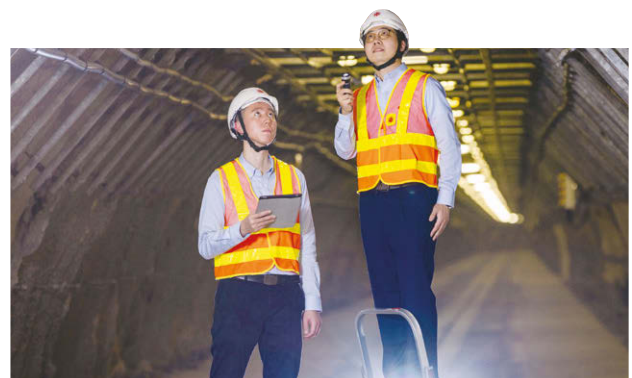
■ Cable tunnels help protect our cables from adverse weather.
