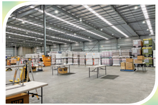
The replacement of lighting with more energy-efficient options in Accensi’s Lara factory helps save energy and reduce our carbon footprint.
