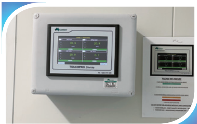
Lipa has installed a dangerous gas monitoring system to ensure the safety of employees in the quality control laboratories.
