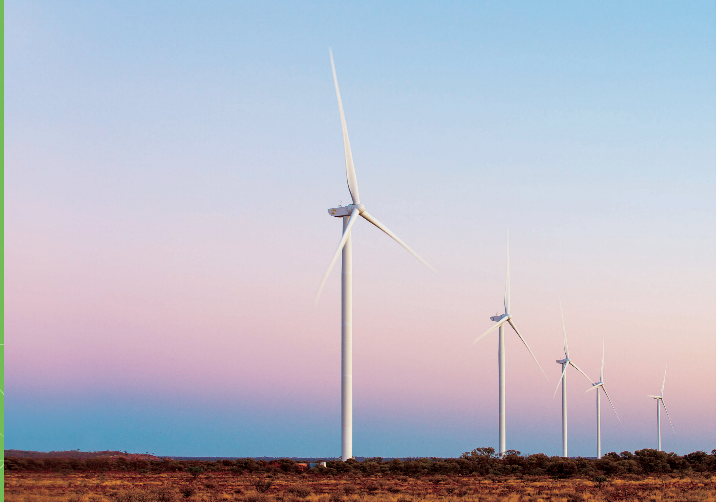
EDL's Agnew Hybrid Renewable Microgrid, a ground-breaking energy solution for Gold Fields' Agnew Gold Mine in Western Australia.
