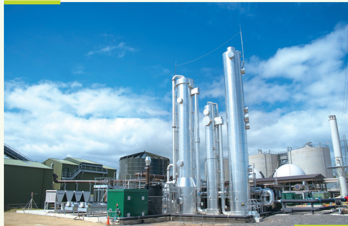
Northumbrian Water aims to achieve net zero in 2027 through innovative practices, including the Organics Ammonia Recovery project that converts recovered ammonia into green hydrogen.
