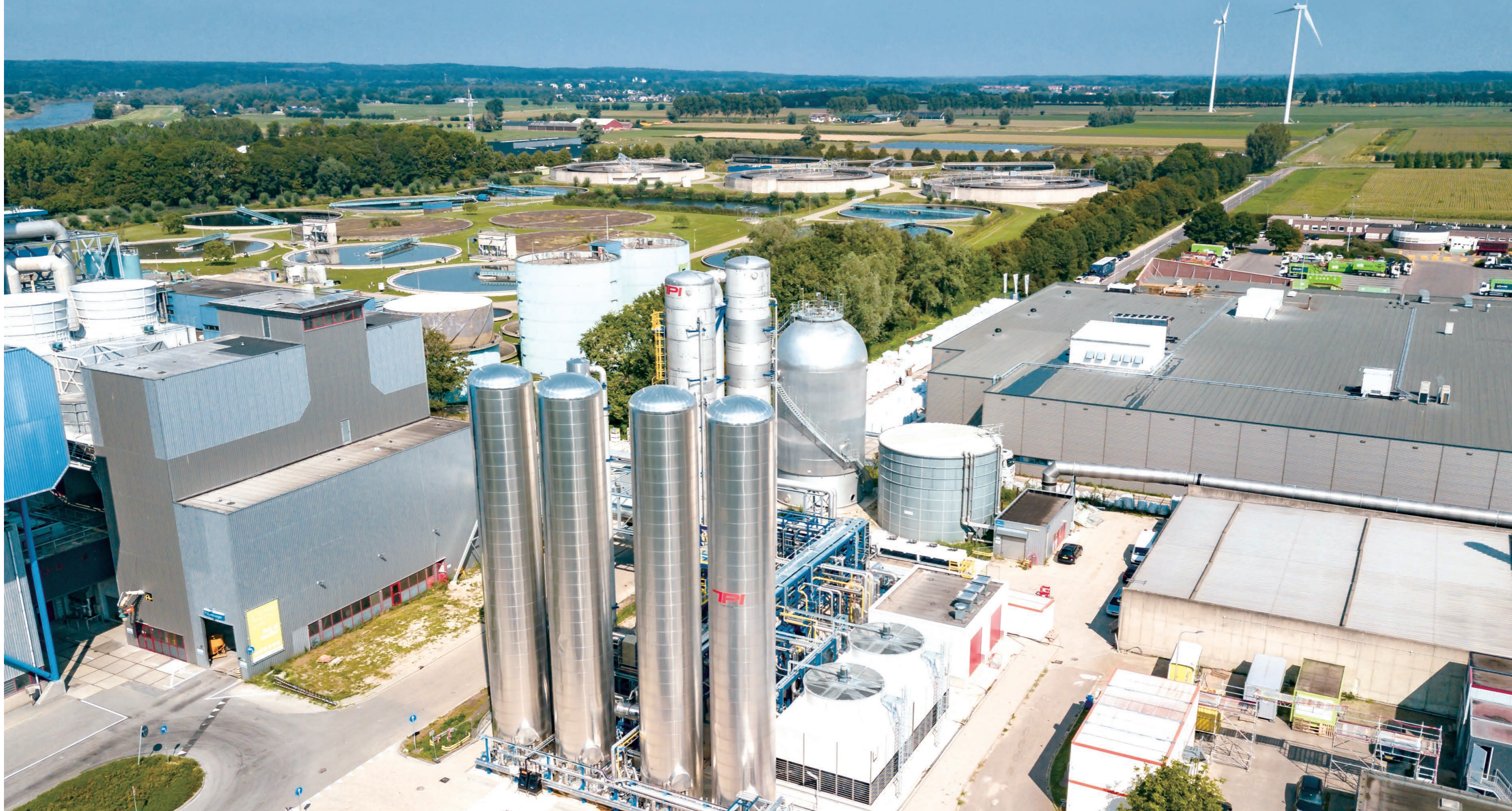
AVR – the CO 2 capture plant in Duiven, used to capture CO 2 for re-use in the greenhouses (Carbon Capture Usage).
