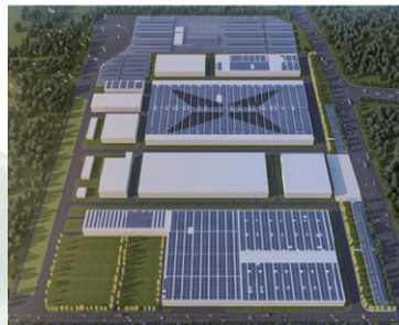
Photovoltaic system of the production base
