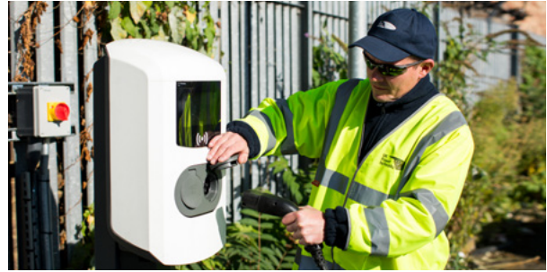
EV charger installation by UK Power Networks
