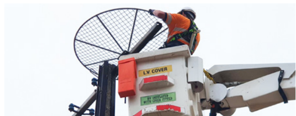
SA Power Networks installing critter guards to protect wildlife
