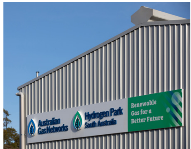
AGIG Hydrogen Park South Australia
