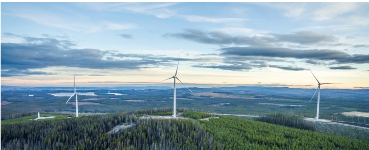
Canadian Power Okanagan Wind farm
