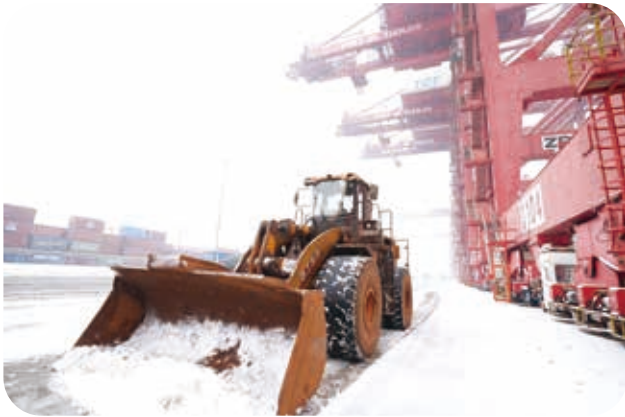
Tianjin Container Terminal cleared the snow in the port area to ensure traffic safety at the terminal apron, the main road, the yard and the rear operating area, thus minimising the adverse impact of snowfall on the safety production of the terminal.
