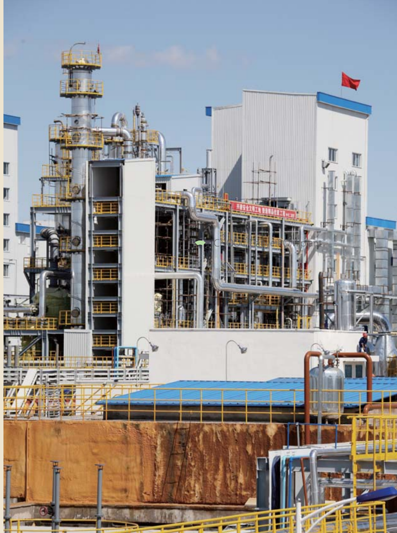
➤ CNOOC Tianye POM plant
