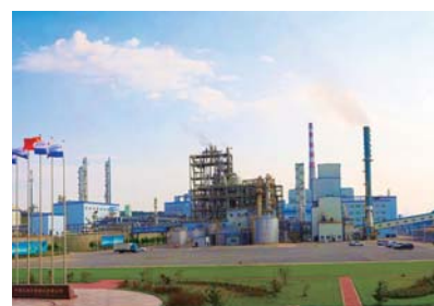
The production facilities in Heilongjiang
