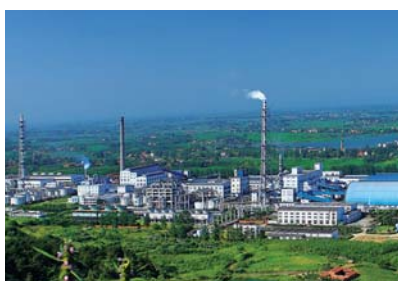
The production facilities in Hubei
