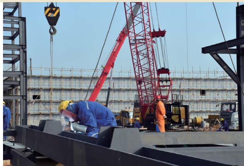
Welding on site
