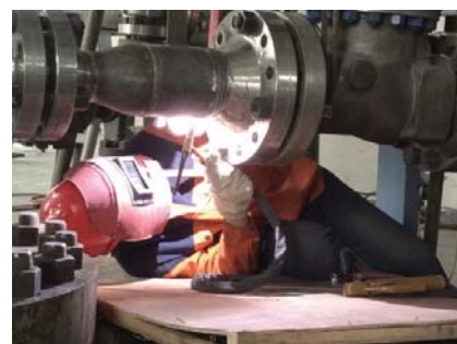
On-site equipment revampment
