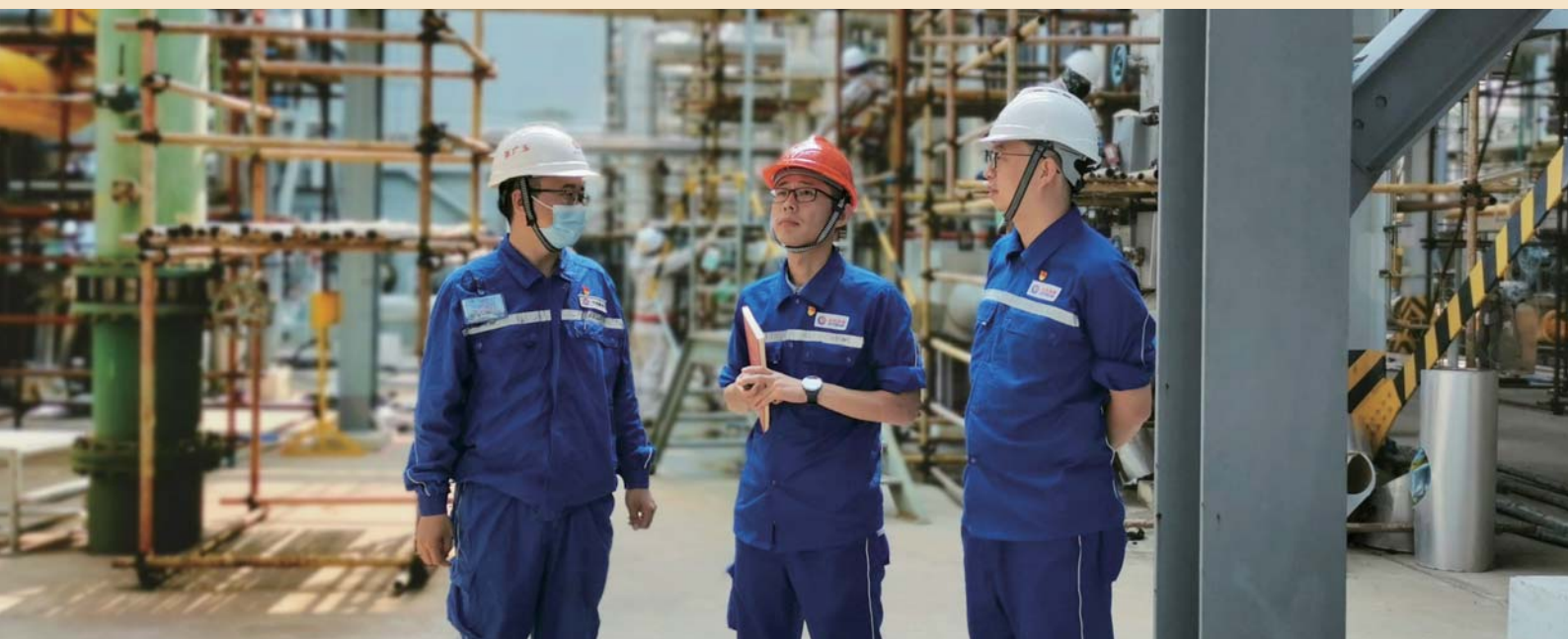
On-site supervision by relevant personnel
