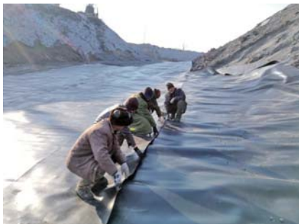
Laying the impermeable membrane of mining pit of CNOOC Huahe
