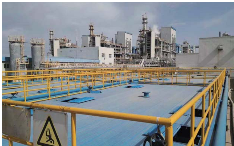
Revampment of sewage system of POM plant
