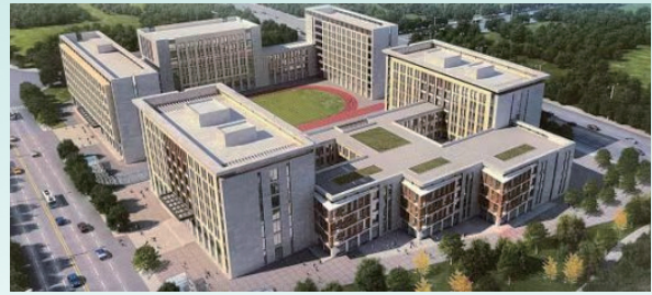
Beijing Municipal Administrative Center C6
