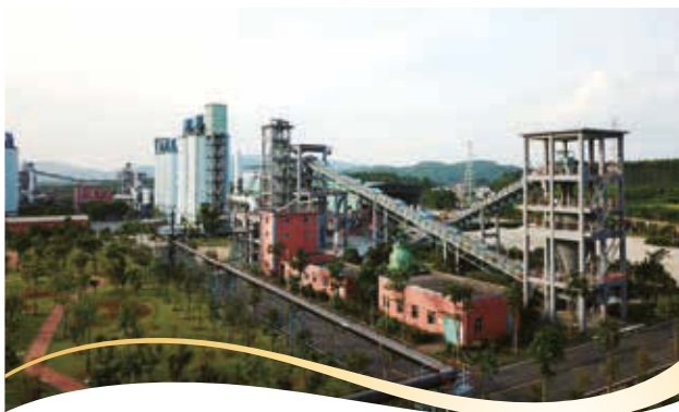
GGBS production plant of Guangdong Shaogang Jia Yang New Materials Co., Ltd in Shaoguan of Guangdong Province
