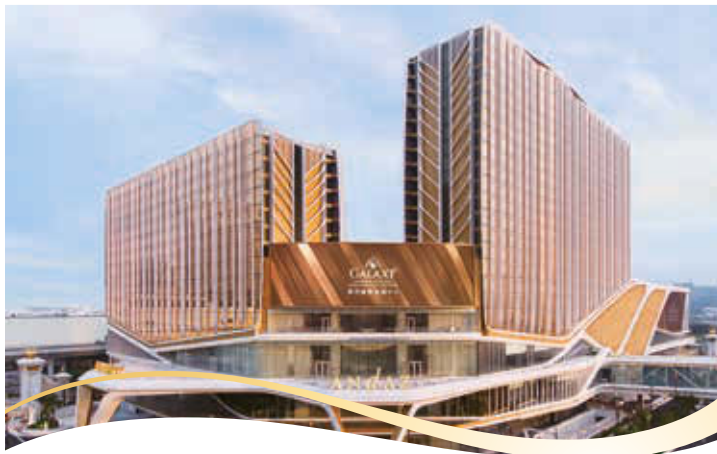
The latest photograph of GICC, Galaxy Arena and Andaz Macau towers
