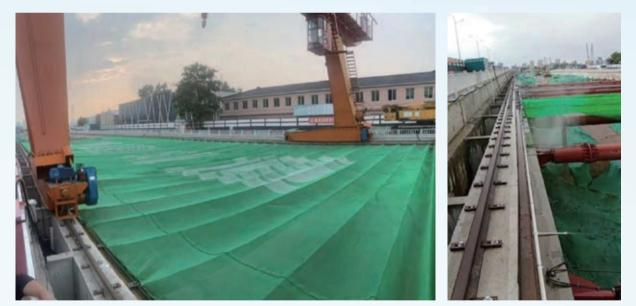
Pictures: Multi-functional and multi-disciplinary electric ceiling (L) Automatic sprinkler system for foundation pit's ring field (R)
