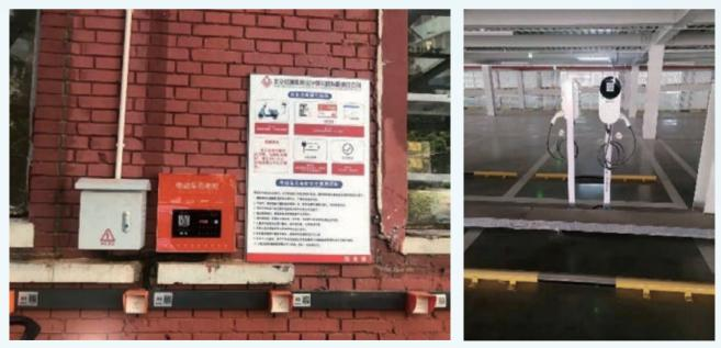
Picture: Electric vehicle charging station
