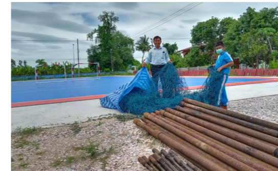
Installing football fence for local schools
