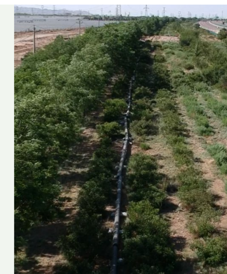
Installing drip irrigation facilities to ensure timely watering of trees
