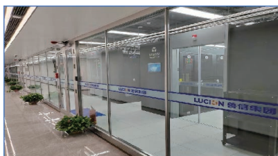
Main data centre (Tower A)
