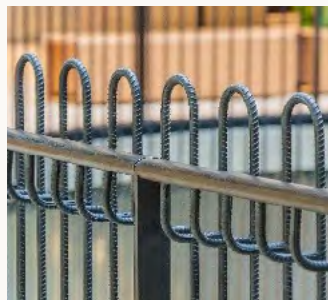
Railing made of recycled steel bars
