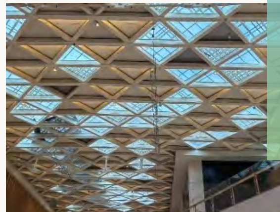
External shading installed at the sunroof of Horizon South and Horizon North in Wuhan Tiandi
