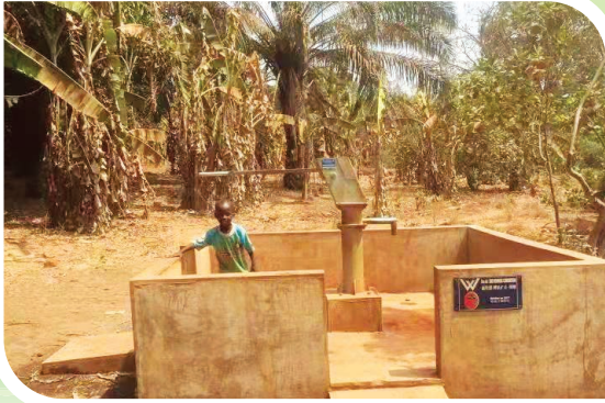
SMB Winning Consortium’s investment in the construction of wells
