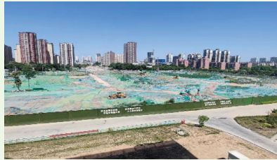
A Photo of Guo Bei Village after Demolition
