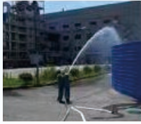
Water Pressure Test
