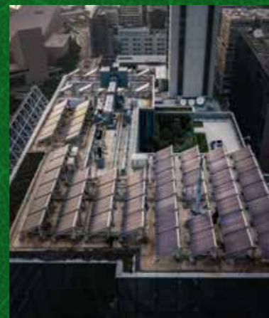
Solar desiccant to control humidity
