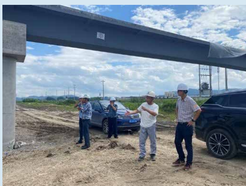
Hazard investigation and correction activity
