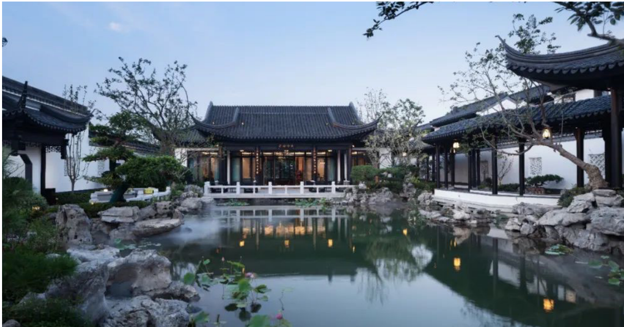
Image: Greentown · Linyi Chun Jiang Ming Yue Project
