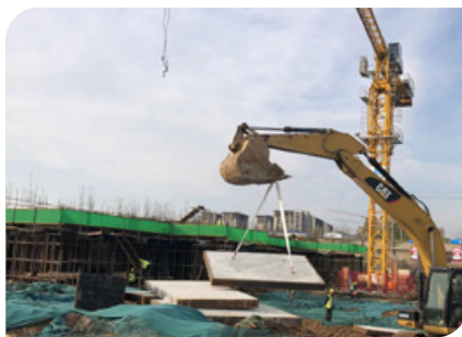
Prefabricated pavement hoisting
