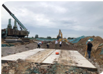
Foundation leveling with a level instrument
