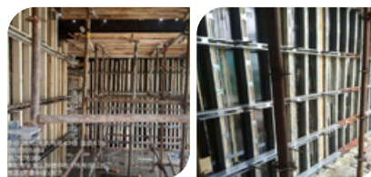
Puyang Sky Mansion Project: Traditional formwork uses a steel reinforcement system.
