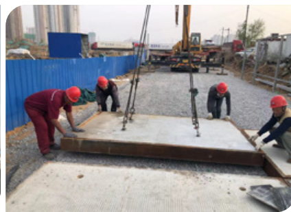
Laying stone cushion layer and prefabricated pavement
