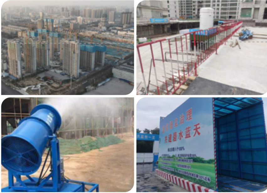
Photos of Xinxiang Xinfei Jianye Mansion's Green Demonstration Project
