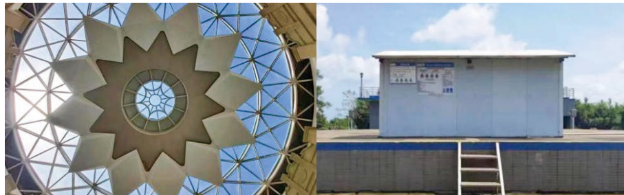
Energy-saving equipment in Terminal 2 T2航站樓節能設備
