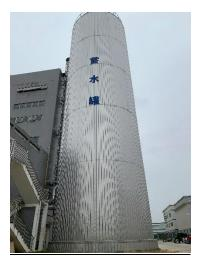
Water Storage Tank – cold energy storage / air-conditioning equipment
