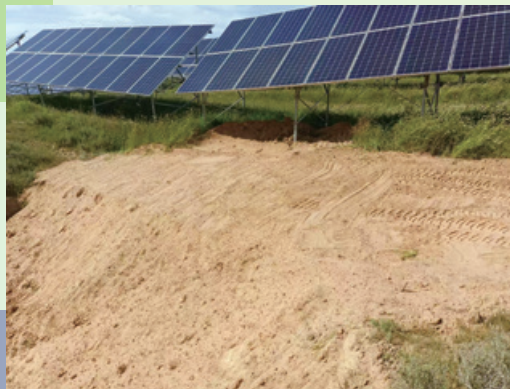
Area 12 After Restoration 12區修復後
