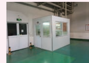
Installation of sound-proofing cabinets
