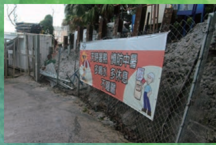
Enhancing the safety awareness of workers by posting posters/banners 通過張貼宣傳海報／橫額，提高工人的安全意識
