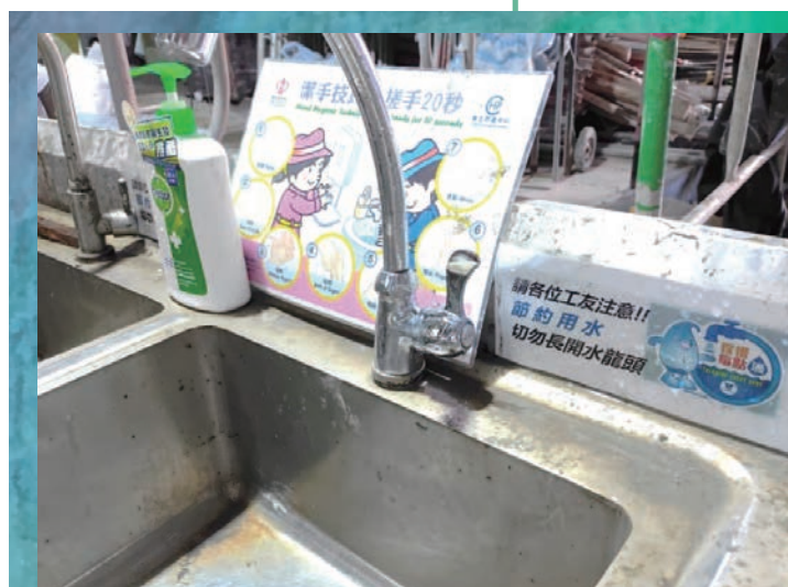
Water-saving Reminder at the Construction Site 施工現場的節水提醒
