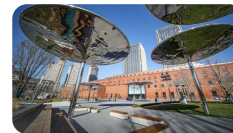
Solar umbrellas at the Riverside Plaza
