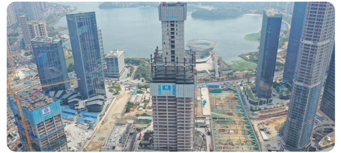
Construction site of Changsha Jinmao Tower
