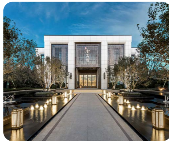
A site of demonstration area of Taiyuan Longcheng Jinmao Palace
