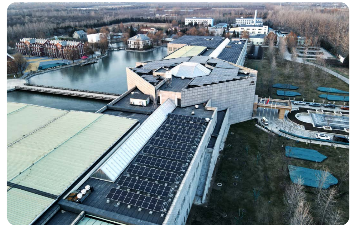
The PV power generation system at Jinmao Eastern Garden Hotel
