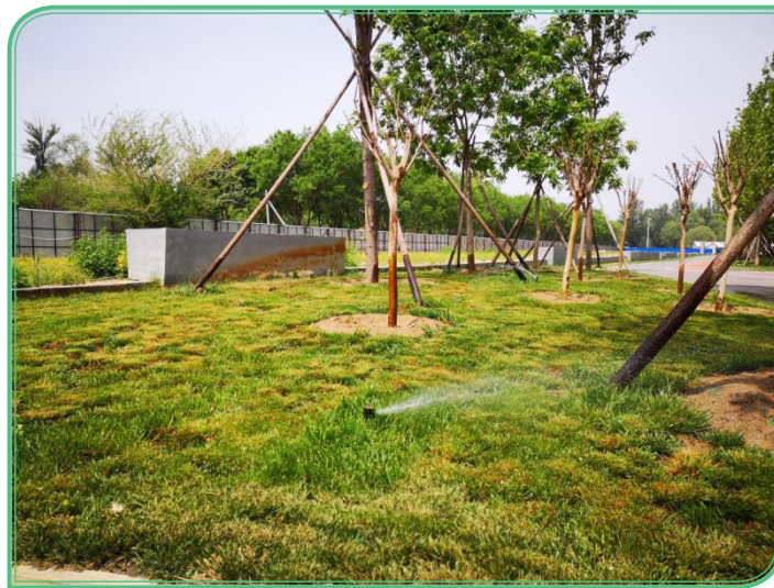
Figure: Green sprinkler irrigation in Houshayu Park
