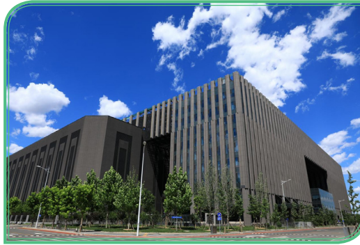
Figure: Houshayu Data Centre of TravelSky
