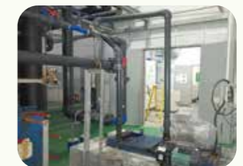
Syringe Pump Modification of Ozone Injection System
