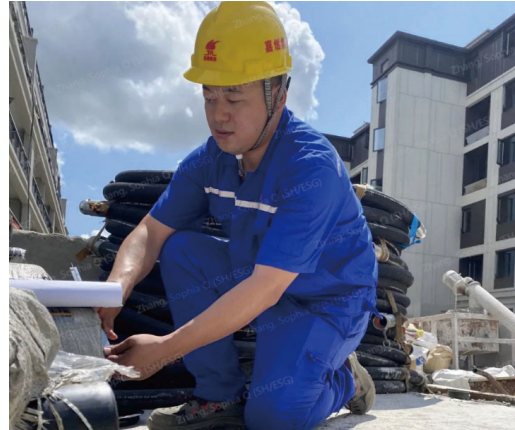
Photo: On-site Pipe Acceptance
