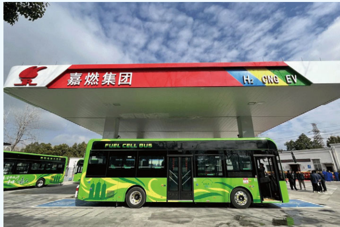
Photo: Gangshan Road Comprehensive Energy Station
