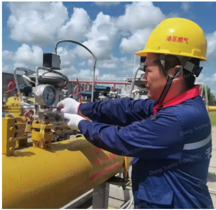
Photo: Staff providing Repair and Maintenance
