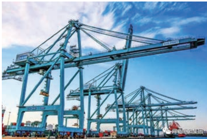
Container terminal in Qinhuangdao Port
