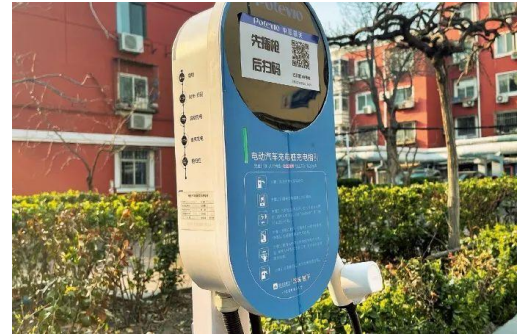
Charging Piles Newly Installed in Old Communities
