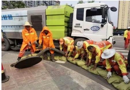
Urban Drainage Pipeline Inspection
