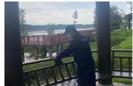
Pre-Typhoon Inspection of Park
