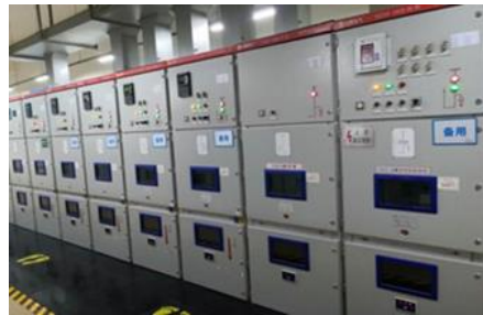
Transformers in Active-Backup Mode
