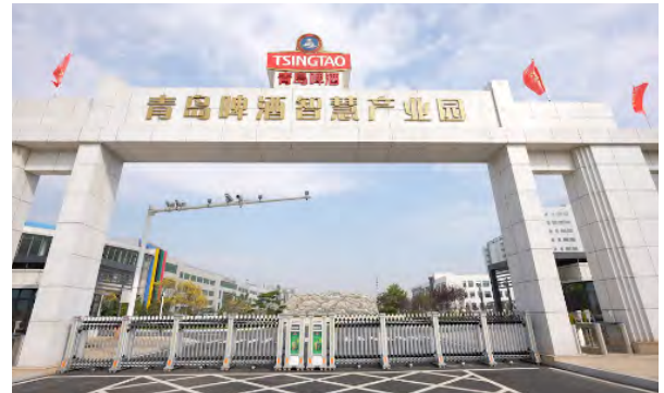
Tsingtao Brewery Smart Industrial Park
