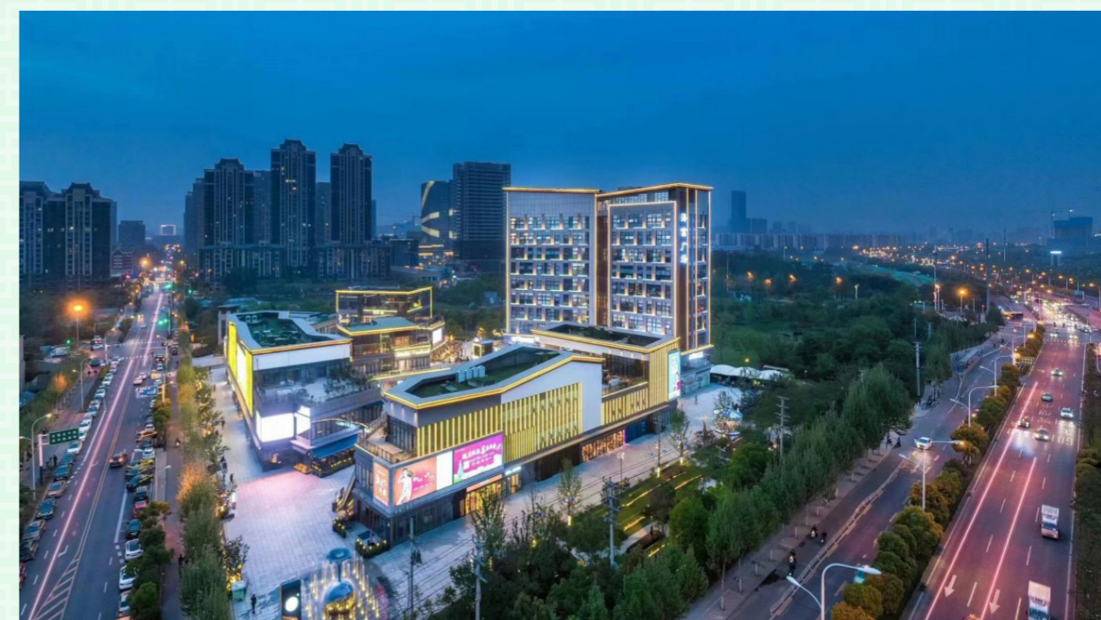
On-site Photo of Hefei Yangshu Huan Yu Tian Di Project
