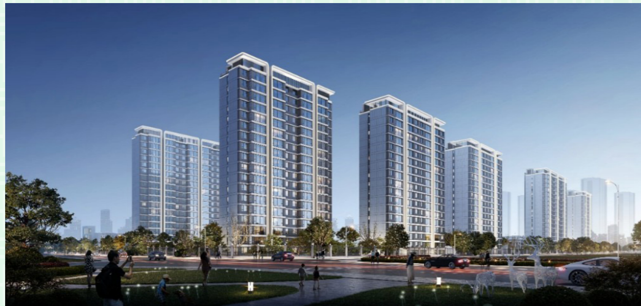
Xuzhou Huayue Project
