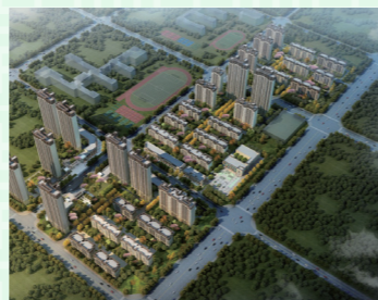
Jining COGO City Project
