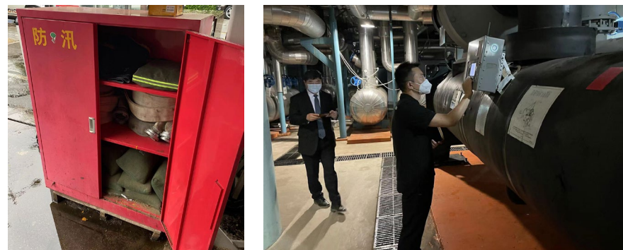
Adequate reserve of flood control Carried out safety inspection
