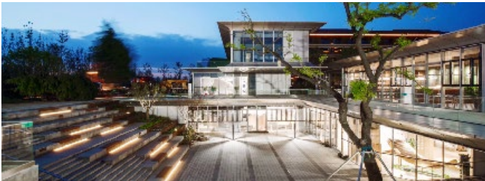
| High Quality Construction Experimental Area (Living) Project
