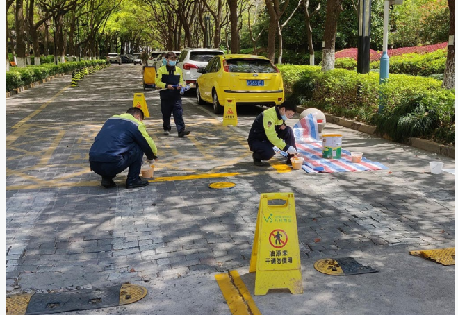
| Road Quality Improvement of Zhongyuan Two Bay City
