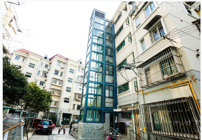
| A Newly Retrofitted Elevator in Shanghai Yangqu Community
