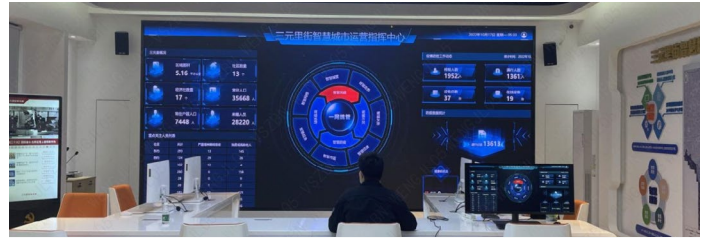
| Intelligent Operation Platform
