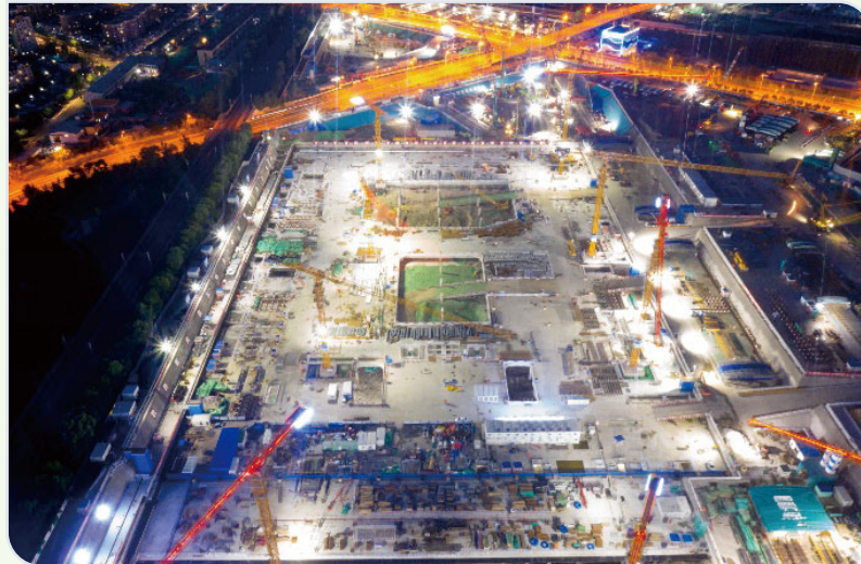
Construction site of Beijing sub-centre station
