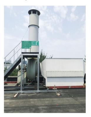
Activated Carbon Adsorption Device
