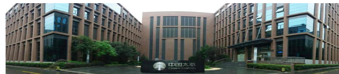
External view of Wuhan Data Center
