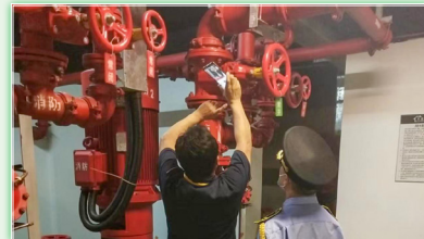
Checking fire pumps
