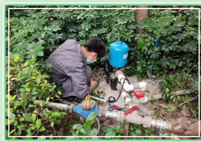
Installing the automatic spraying device
