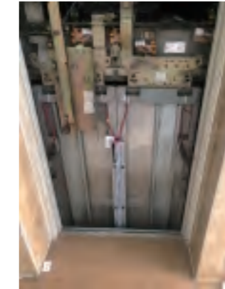
Installation of light-screen electric vehicle resistors
