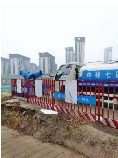
Dust suppression devices installed at various spots on site
