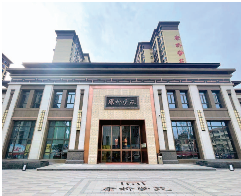
The Xixian Kangqiao Xueyuan project in Henan Province
