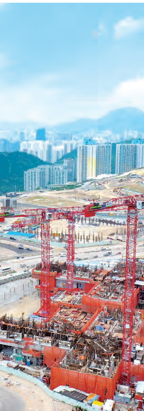
□ Construction activity proceeded on track
