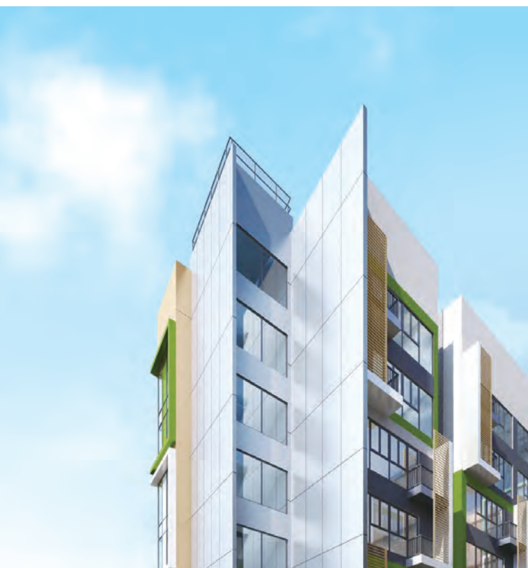
□ The Multi-welfare Services Complex in Kwu Tung North is the Group's first project with full MiC application
