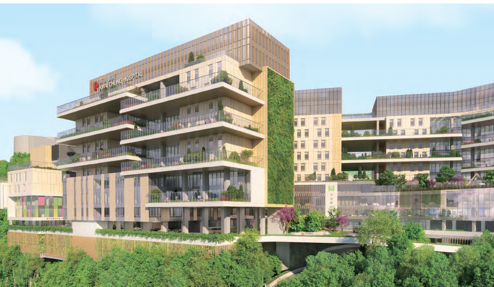
□ The redevelopment of Kwai Chung Hospital Phase 2 is in good progress
