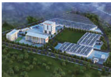
Photovoltaic power generation system on the rooftop of the plant 廠房屋頂佈置光伏發電系統
