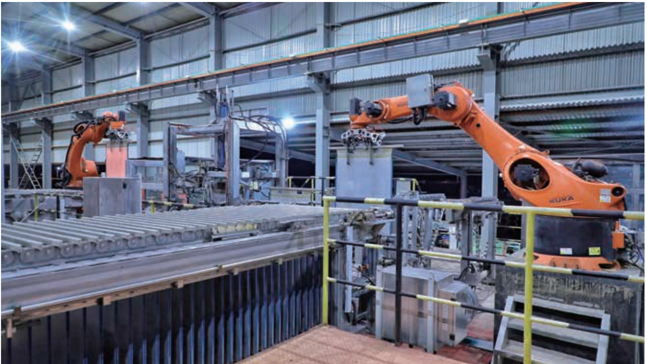
Copper cathode stripping operation in the electrowinning workshop of the Kambove Mining Leach Plant
