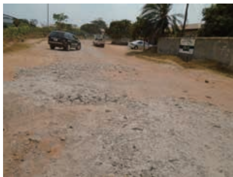
After paving the road with gravel
