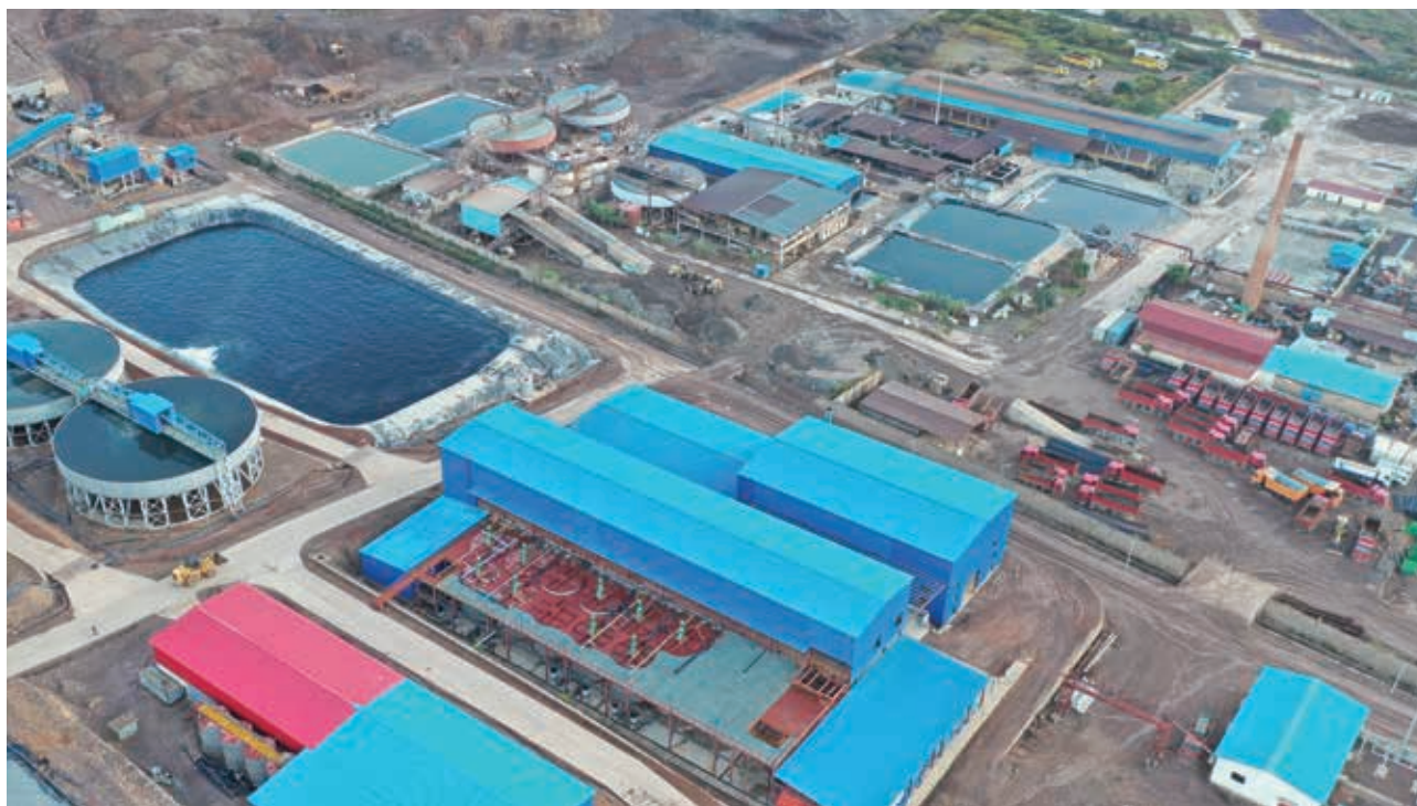
General view of Huachin Leach
