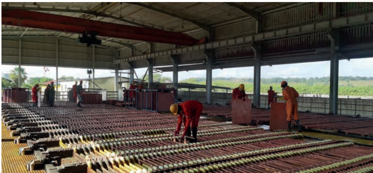
Chambishi leach extraction and electrowinning workshop production site
