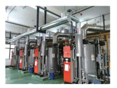
Low-nitrogen burners used for the gas-fired boilers in Beijing plant
