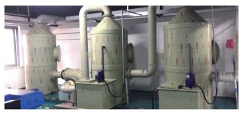
Harmless treatment of exhaust gases used for the sewage treatment system in Beijing plant
