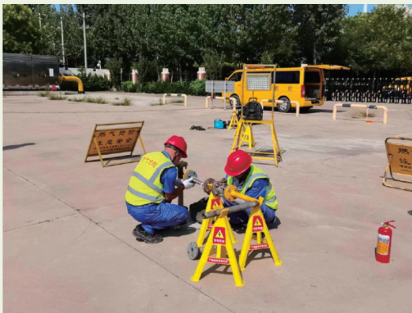
Photo: The Emergency Repair Drill Site
