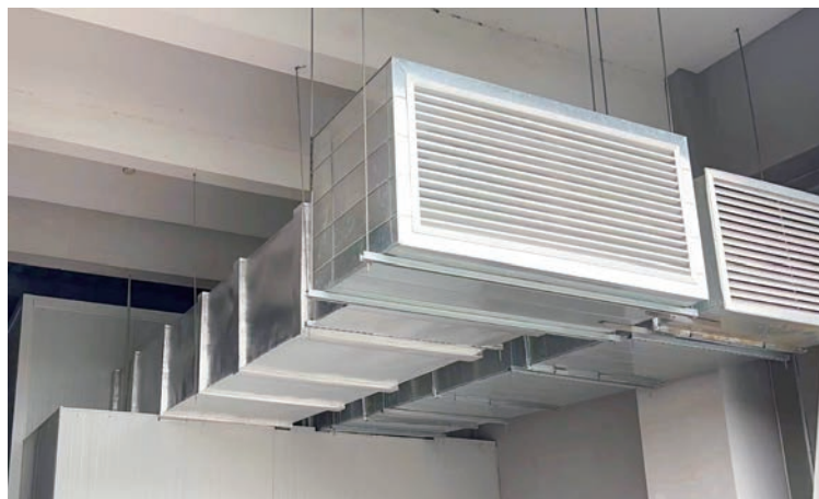
Sound insulation measures for air compressors in Shanghai Zhoupu Park
