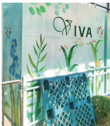
New water treatment facilities in Faladi Road Park
